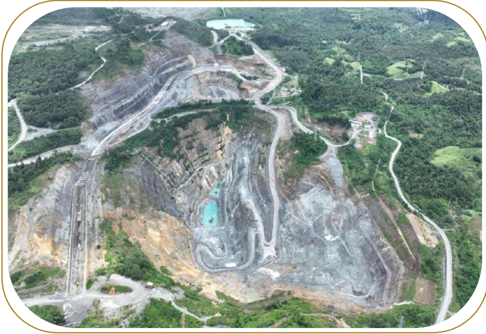
Pit condition before Natural Disaster (March 2024)
