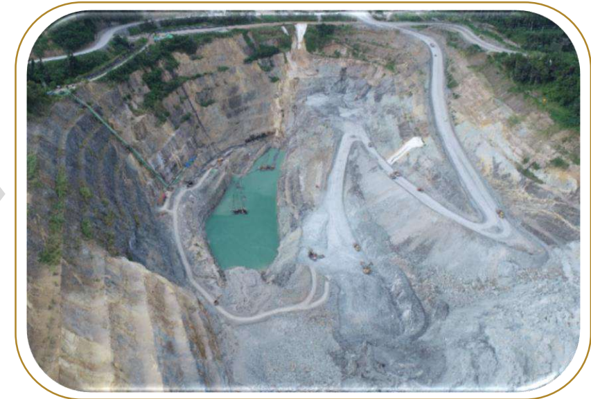
Pit condition per July 2022
